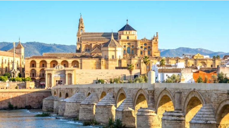
Historic Centre of Córdoba
